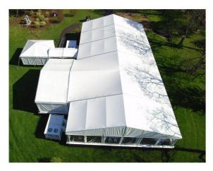
The Aluhall ranges from 3m in width to 25m and is extendable in 3m or 5m bays.
